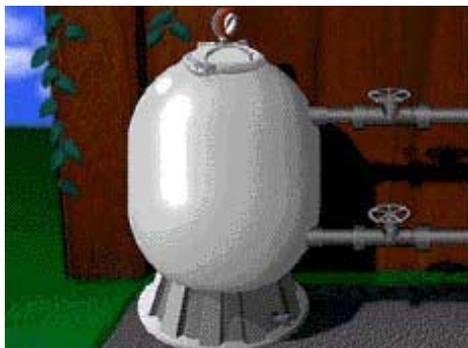
The filter is one of the most important pieces of equipment in a pool. A clean, properly functioning filter removes debris you can see as well as some you can't see. Pool water that is not filtered properly can appear dull and cloudy. Debris places demand on the sanitizer, making it hard to balance and maintain proper pool chemistry. There are three kinds of filters pool owners might use:
